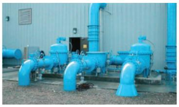
Eaton automatic strainers provide filtration of incoming water protecting membrane system in rigorous application including seasonal algae bloom.
